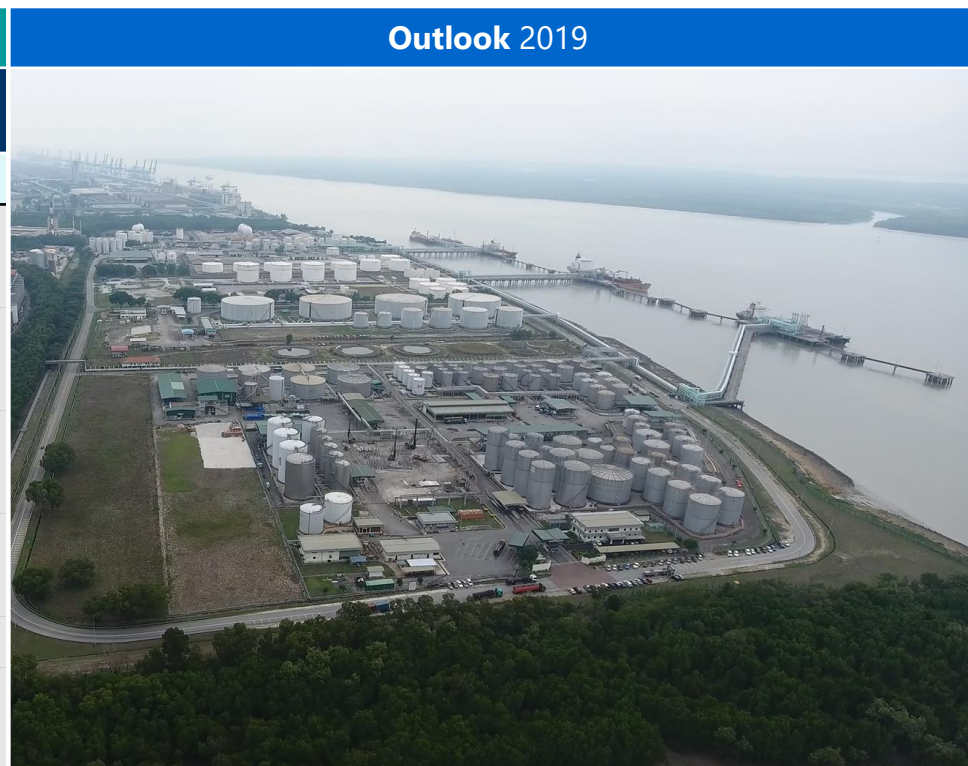
Westports to build additional jetty to support the long-term growth at Liquid Bulk operations
