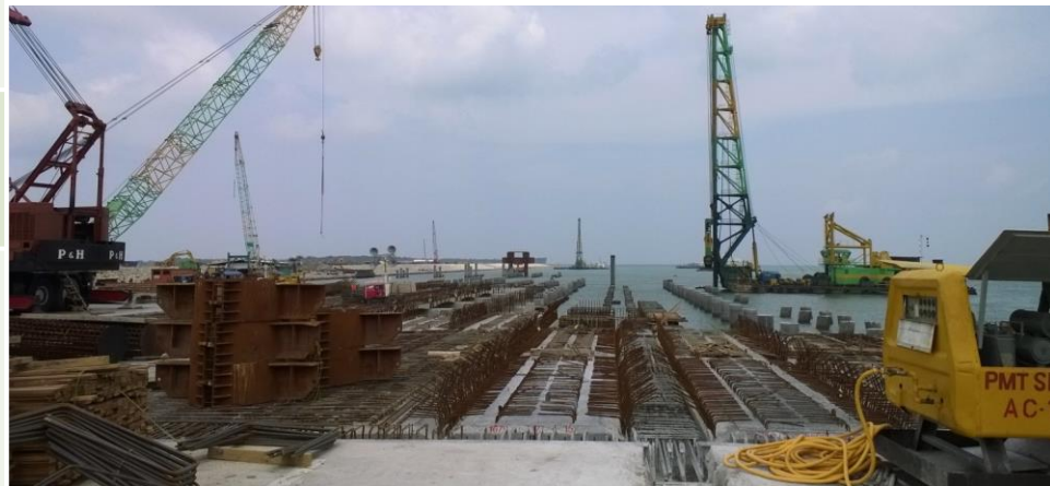
▲ Concrete wharf surfacing for first 150-metre is completed ▼ June 2015 Casting of wharf deck
