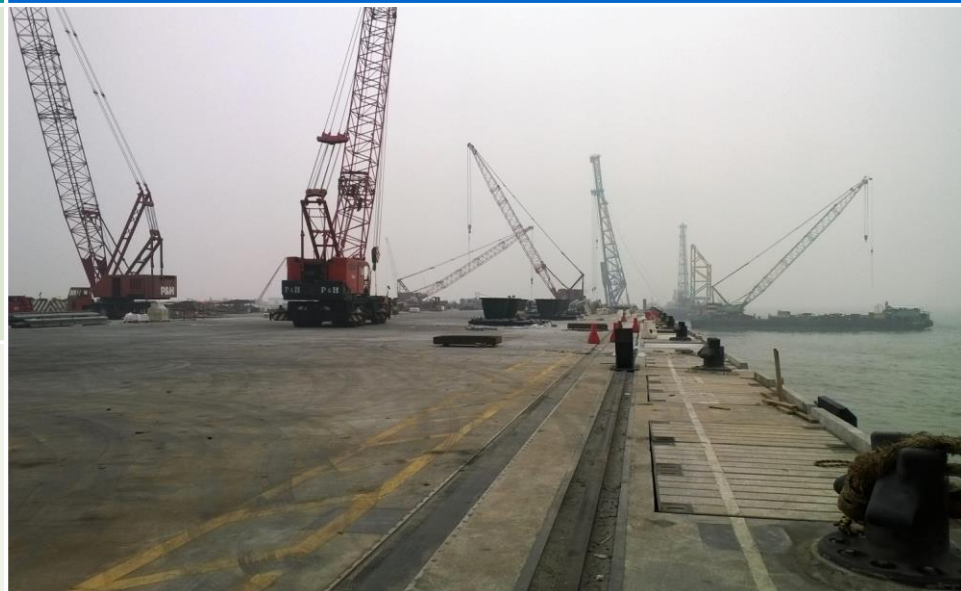
▲ Concrete wharf surfacing for first 150-metre is completed ▼ June 2015 Casting of wharf deck
