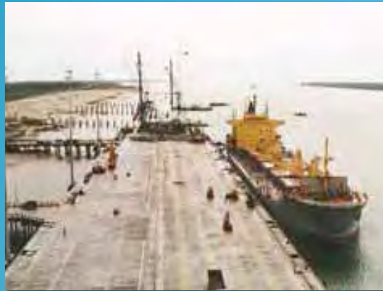
First 600m berth being constructed
