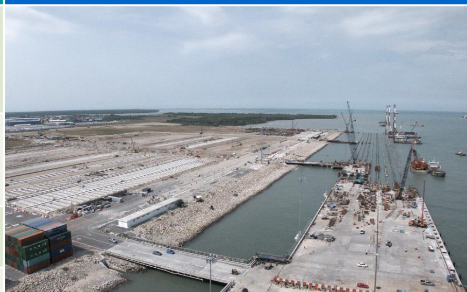
CT8 Phase 2 300-metre wharf is near completion. Advanced progress with CT9 piling
