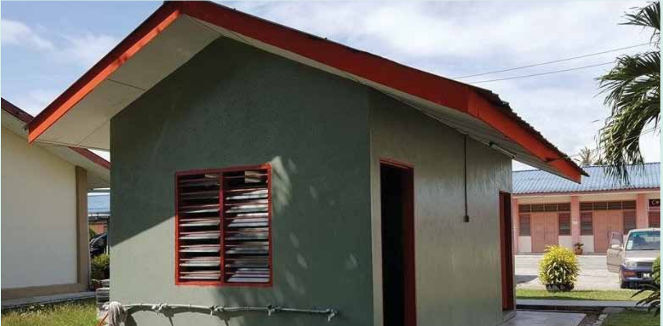
The result of the effort by the Engineering department is a better toilet facility for the use of the children, teachers and staffs of Kafa Integras Kampung Perigi Nenas, Pulau Indah
