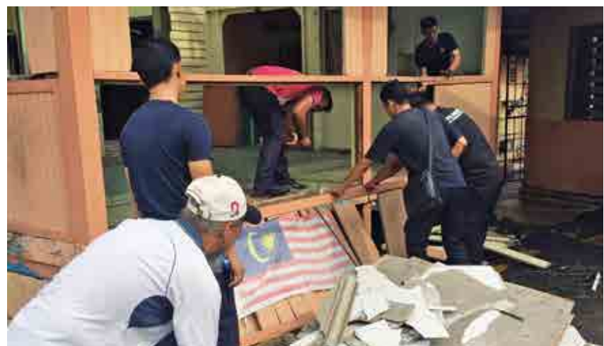
▲ The Engineering Team helped refurbish the surau in a kampung on Pulau Indah as part of its CSR activities.
