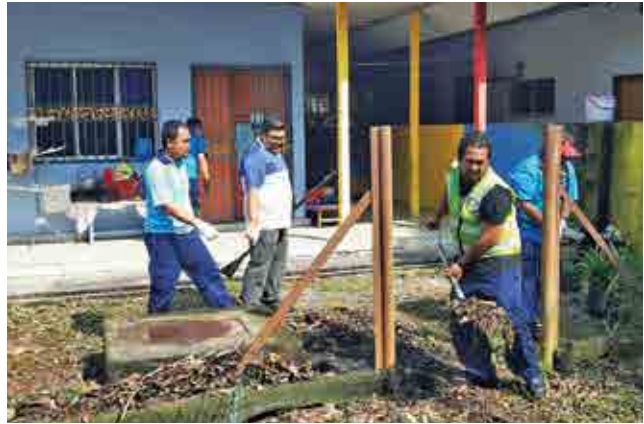
▲ As part of its contribution to the local community, two houses in Pulau Indah were refurbished by the Engineering Team to help ensure the safety and well-being of its occupants.
