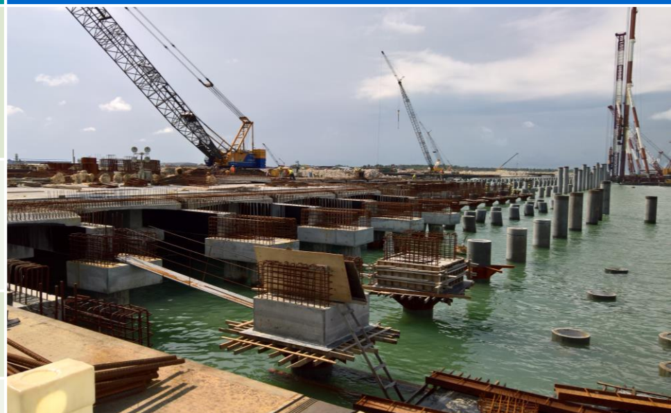
Prestressed beam and ongoing concrete works for CT8 Phase 2 300-metre wharf
